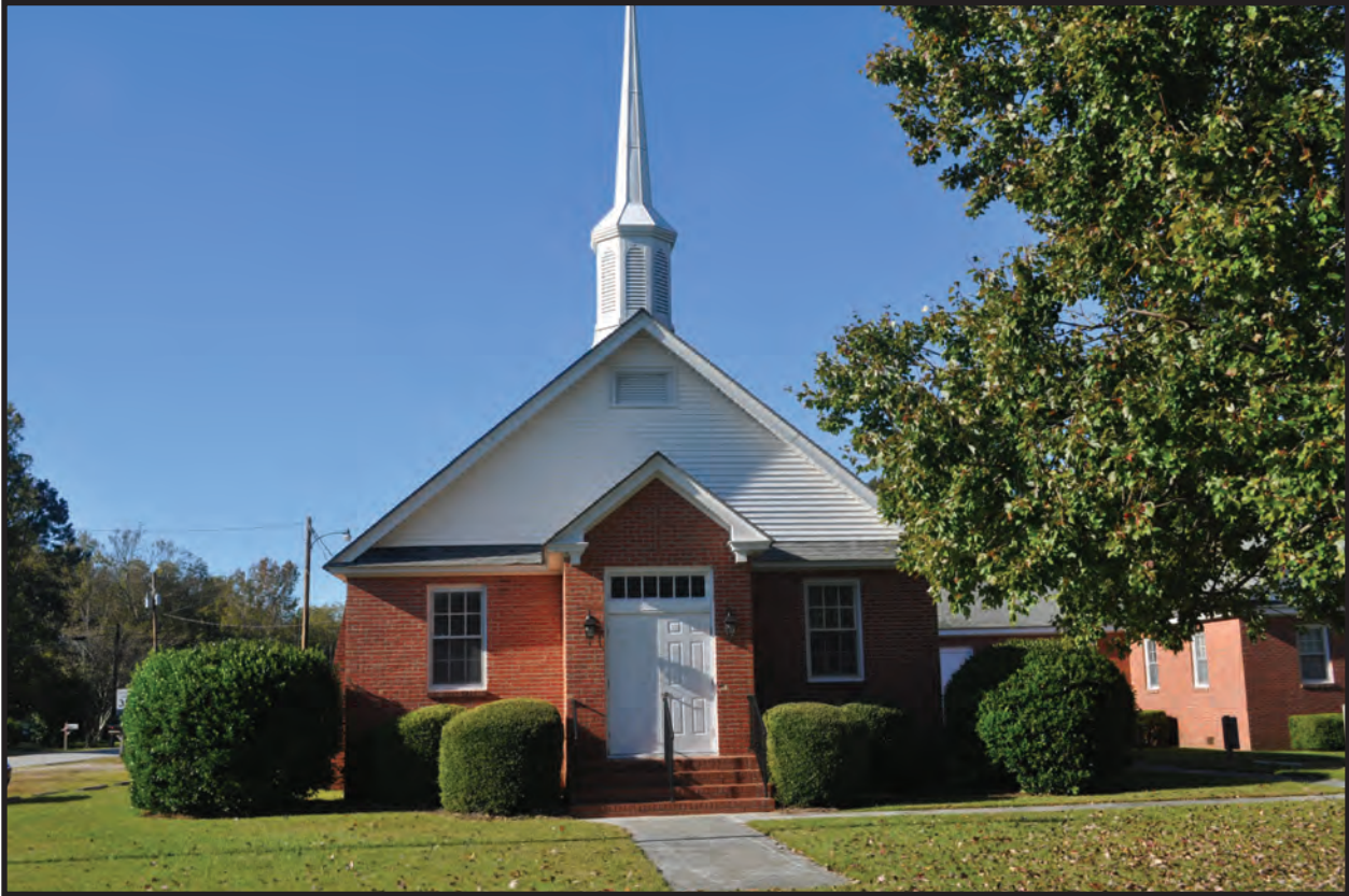
Figure 72. Neuse Forest Presbyterian Church Sanctuary, Northeast Side
