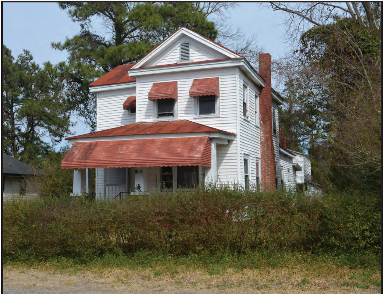
Figure 44. Dudley House Front/West Side
