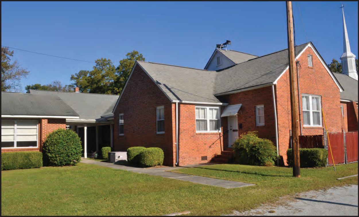
Figure 73. Neuse Forest Presbyterian Church Sanctuary, Southwest Side
